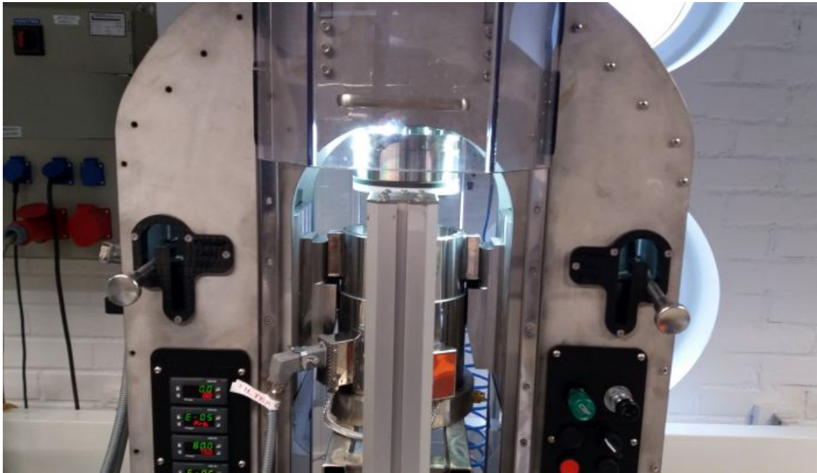
Figure 9 – Installing the filtration unit
